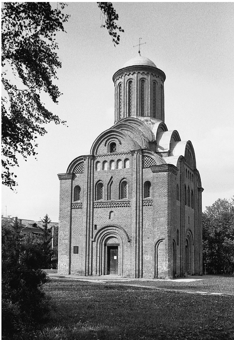
Figure 11 The reconstructed Church of St. Paraskeva Pyatnitsa, Chernigov
